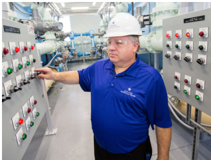
Removing iron from the source through filtration
