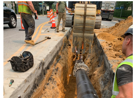
Replacing aging pipes
