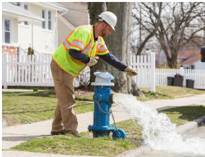
Flushing our pipelines
